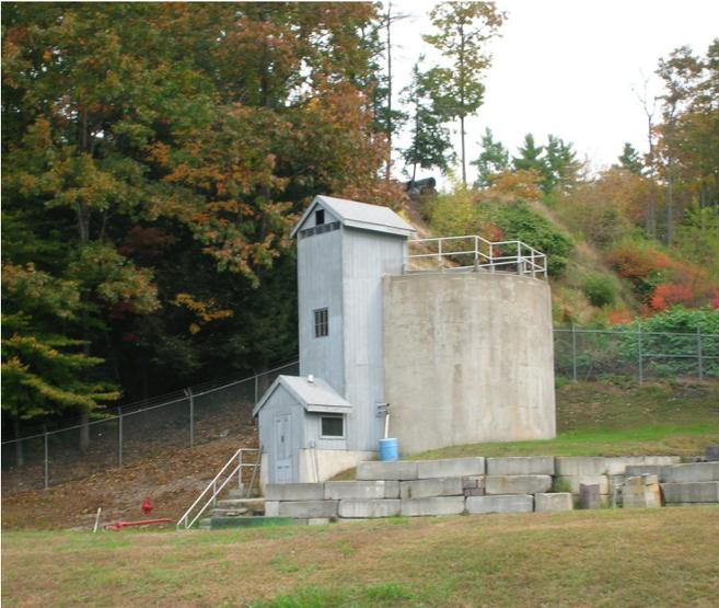
**Shown here is the 60,000-gallon aerated sludge holding tank that will have a new VFD controlled blower motor.**
