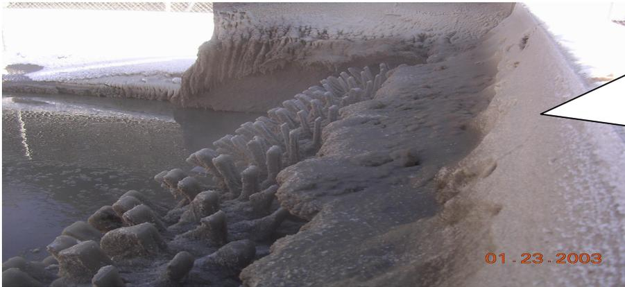
**The frozen Rotor on the Oxidation ditch prior to the development and installation of the Heated Splashguard**
