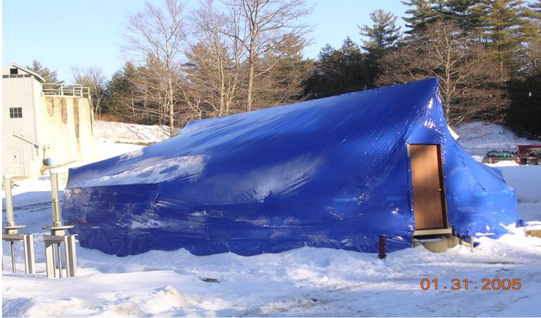
This photo shows the large clarifier with a cover made with boat shrink-wrap the framing was done by facility staff and the cover was put on by West Shore Marine with the help of Wild Horse Welding's boom service. The cover protects the clarifier from freezing in the winter as well as preventing the growth of algae in the summer. This cover will be replaced with a more permanent cover during our 2008 facility upgrade.
