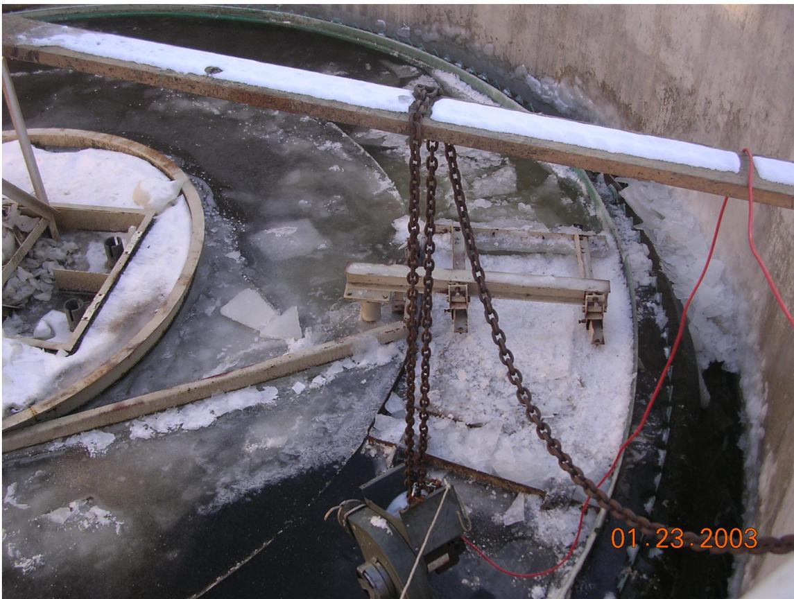
This is the frozen clarifier prior to the installation of the shrink-wrap cover. Ice would form at times up to 1 inch per hour on the surface. The staff would need to
