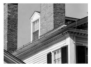
Example: Gutters constructed of wood, seamless painted aluminum or other metal will be approved if their scale, contour, and detail are found to be compatible with the style of the building.
