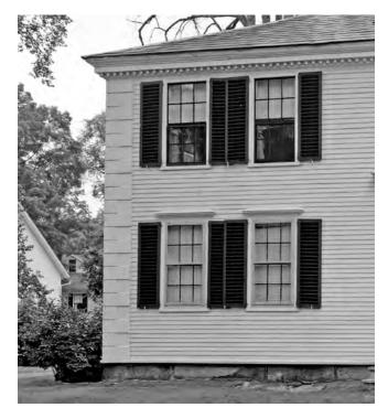
Example: Functioning shutters—wood louvered and paneled shutters, installed on shutter hinges with retaining "dogs" lag-bolted to the exterior wall. The size of the shutter should be equal to the height of the window opening and one-half its width.
