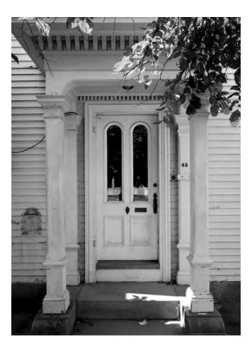
Example: Wood doors should be constructed in a manner consistent with their traditional manufacture: assembled of stiles and rails, with an infill of wood panels and/or glass lites.
